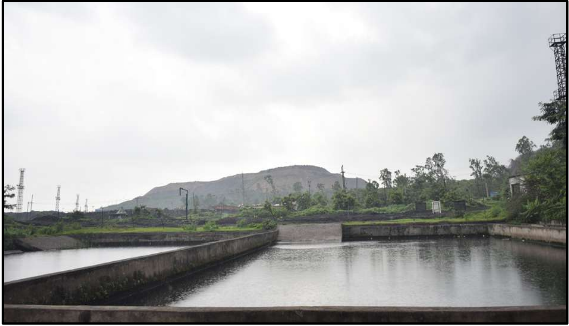
Sedimentation tank at MDTP, Iajkura OCP
