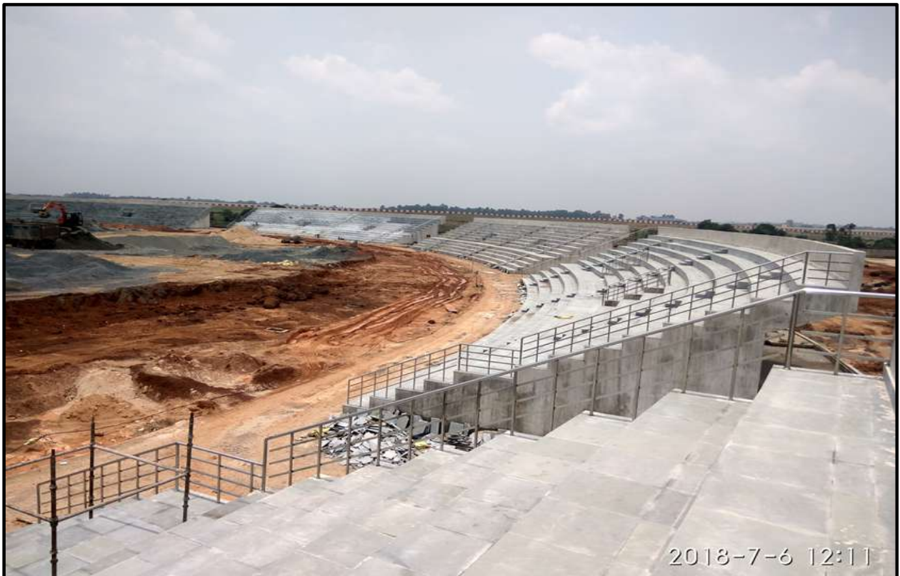
Stadium under construction at Jharsuguda
