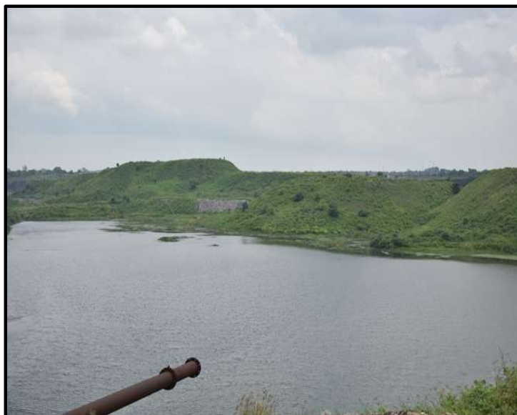
Water harvesting structure at Hingula OCP
