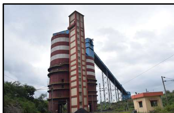
Silo at Bharatpur OCP
